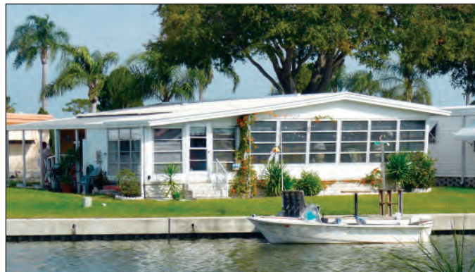
Seawalls can help minimize shoreline erosion but may cause other problems.
